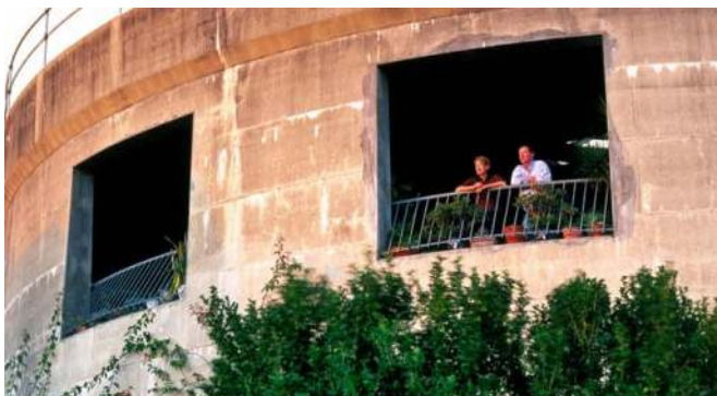
Tank house on the hill at Balmoral, Australia
